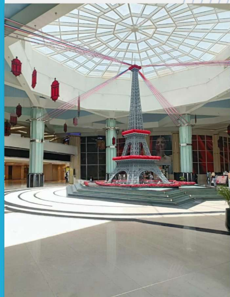
Metal Frame with Acrylic skylight
